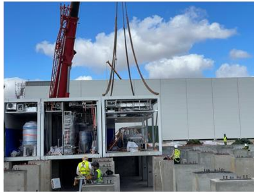
Module lifting
